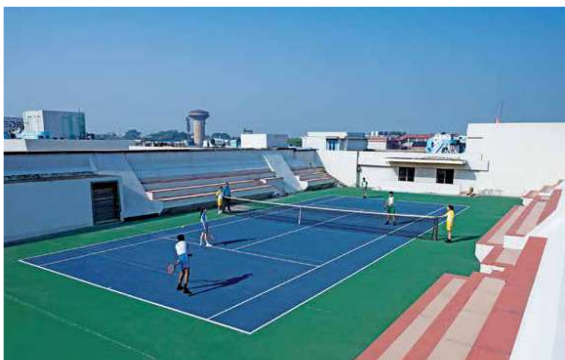
ROOF-TOP 'WIMBLEDON' STYLE TENNIS COURT
